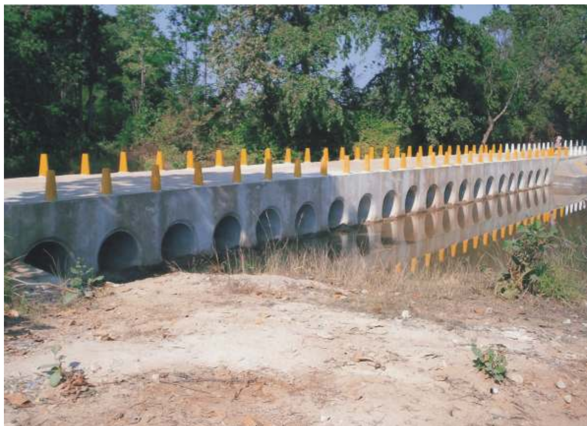
Vented Causeway at Naharbagicha, Block- Bamra, distt. Kuchinda, Orissa, constructed with the Article 275(1) funds.
