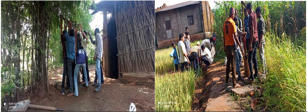
Youth Repairing Community Hand pumps
